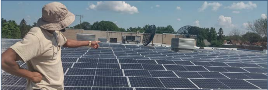
NORTH COMMUNITY HIGH SCHOOL | MINNEAPOLIS, MN | CREDIT: MINNESOTA RENEWABLE NOW
